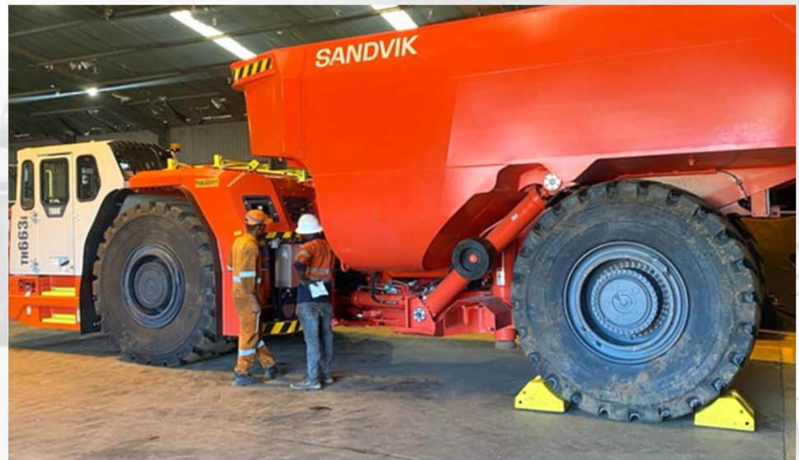
WORK DONE - ASSEMBLING SANDVIK UNDERGROUND TRUCK.
