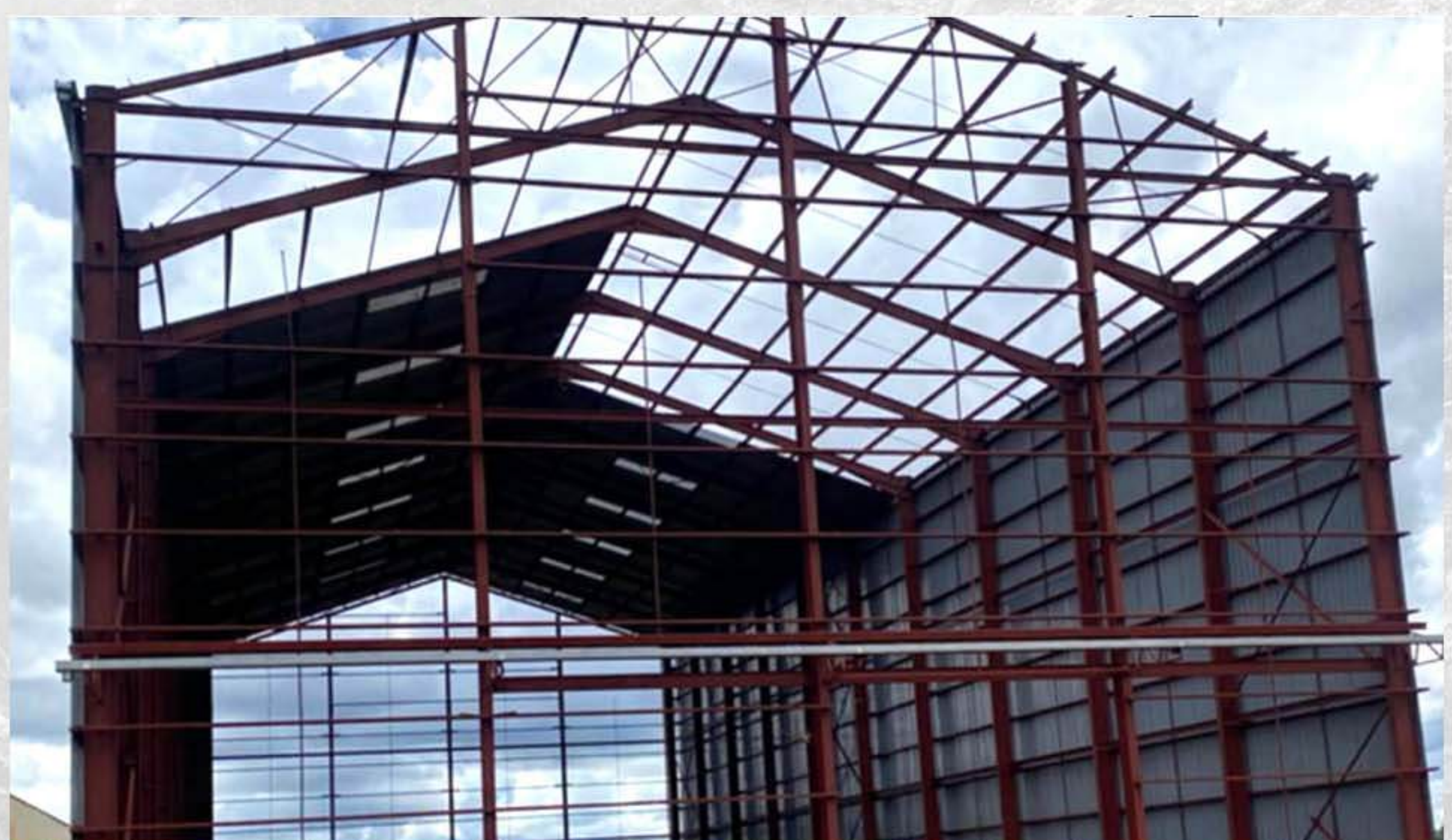
NEW WAREHOUSE UNDER CONSTRUCTION - DESIG- NATED NEW STORAGE FACILITY.
