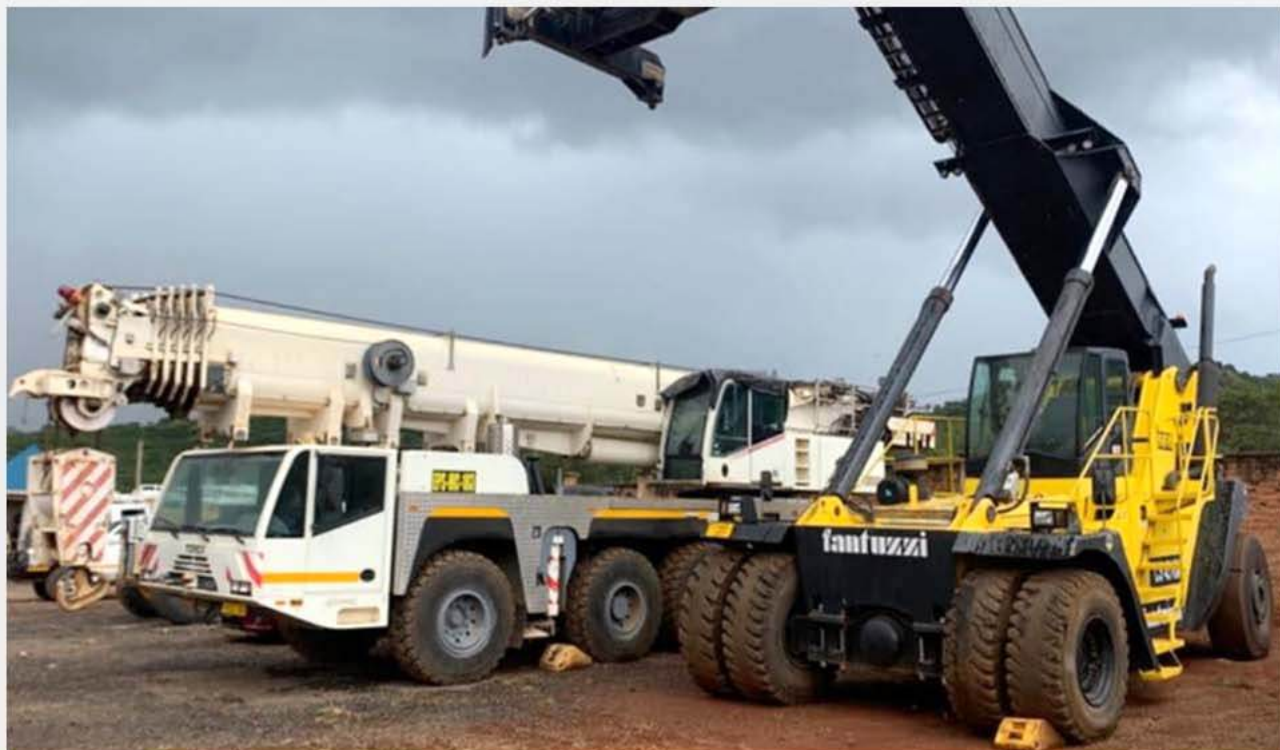
LIFTING/RIGGING EQUIPMENT 140 TON TEREX CRANE, 45TON FANTUZZI REACH STAKER.
